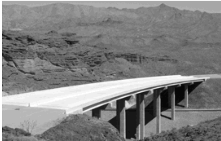
View of new U.S. 93 alignment as it crosses the Sugarloaf Mountain Bridge.
