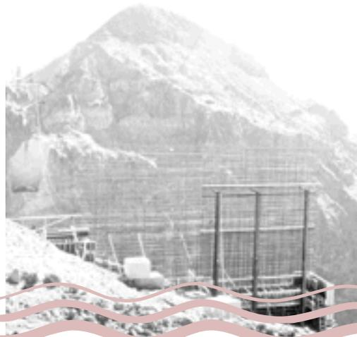
View from the Nevada side of the Colorado River Bridge alignment looking east toward Arizona. In the foreground, formwork is being constructed and reinforcing steel is being placed for the Nevada bridge abutment.
