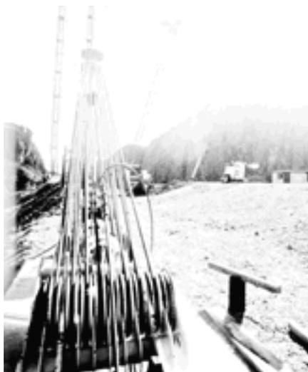
*A view of the south tower crane's twin, 14-part pulley system. The pulleys apply tension to the twin, 3-inch high-line cables that span the canyon.*
