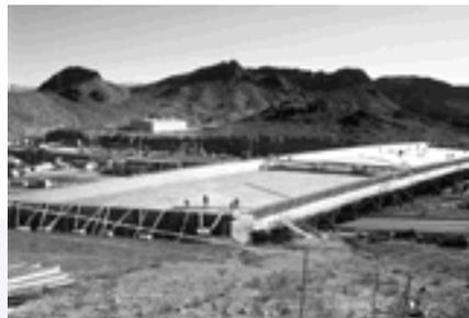
*Edward Kraemer & Sons crews construct formwork and place reinforcing steel on the Bureau of Reclamation Warehouse Bridge.*
