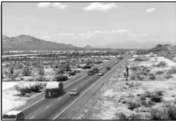
Level of Service B.
