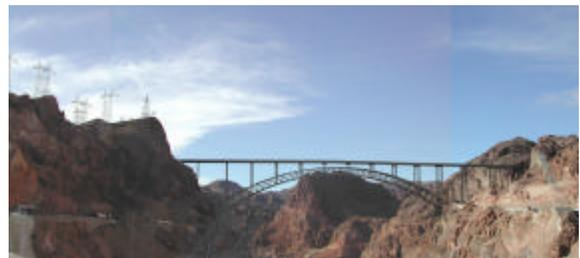
erection methods, high strength steels and high strength concretes, the trussed arch rib and suspension spans were the only alternatives considered for spans in this range. The proposed structure consists of a 1325-foot main span arch with 455-foot and 235-foot approaches on the Nevada and Arizona sides of the river respectively, for a total structure length of 2015 feet. The variable depth trussed-ribs are vertically oriented with parallel and vertical spandrel columns. The
