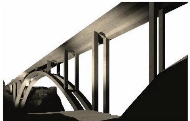
3. **Concrete – Steel Composite:** The concrete composite alternative combines a twin rib concrete arch with steel spandrels and a conventional steel box girder with
