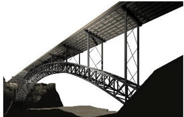
The superstructure is comprised of steel plate girders spanning approximately 130 feet with a composite concrete deck. The approach spans are similarly comprised of vertical column bents supporting a steel plate girder superstructure with spans to 160 feet. The vertical and diagonal web members of the trusses will be structural tubing. All bent and rib bracing members will be also fabricated from structural tubing.
