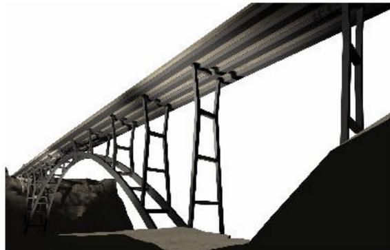
2. **Concrete Solid Rib:** This concrete alternative is a classical twin rib concrete arch, with cast-in-place spandrel columns, and a cast-in-place concrete box girder deck.
