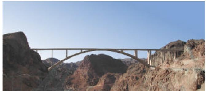
for the long span alternative. The spandrel columns are also concrete, and assumed to be cast-in-place. Precast segmental columns may be considered, depending upon the capacity of erection equipment. The deck system is similar to the short span solid rib concrete, being a twin box girder structure.
