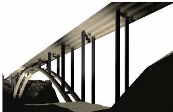
4. **Steel Viereendeel Arch:** The Viereendeel-rib alternative is an option that was devised
